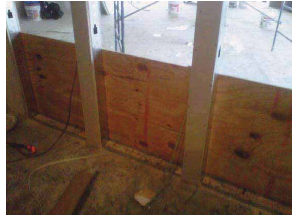
OUTER 5/8 PLYWOOD WALL (to match thickness of outer sheetrock)
