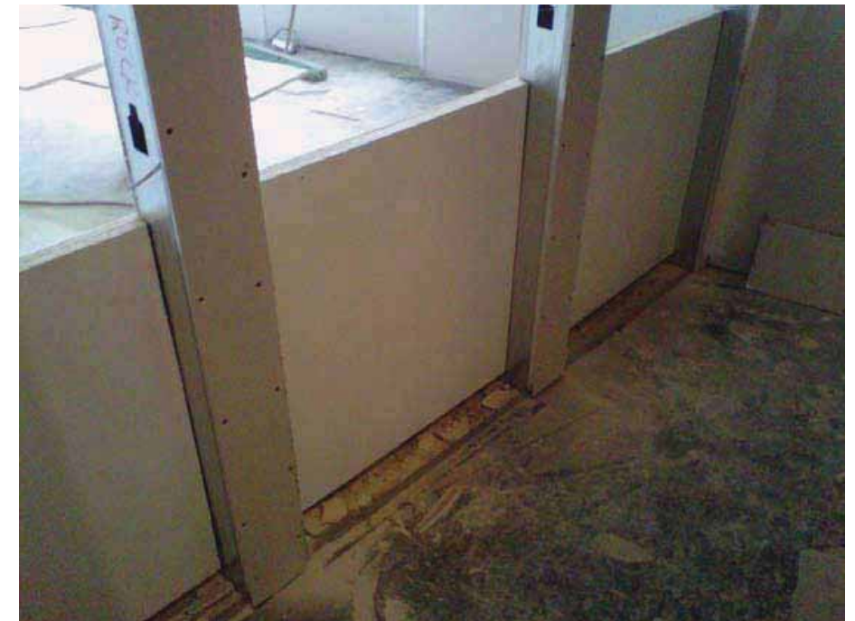
INNER FINISHED 3/4 MELAMINE, STUDS TO BE WRAPPED WITH FRP
